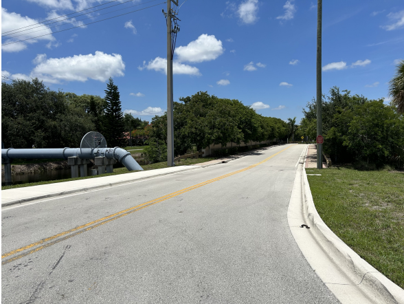
Phase II (Entrance Road) (3)
