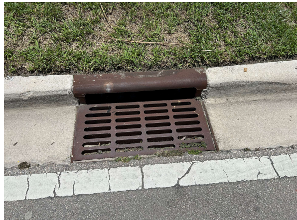
Phase II (Drainage Inlet) (6)
