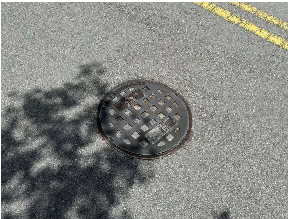
Phase I (Sanitary Sewer Manhole) (25)
