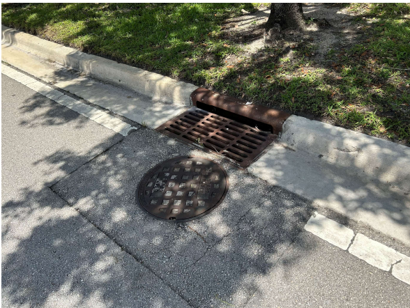
Phase I (Drainage Inlet) (5)
