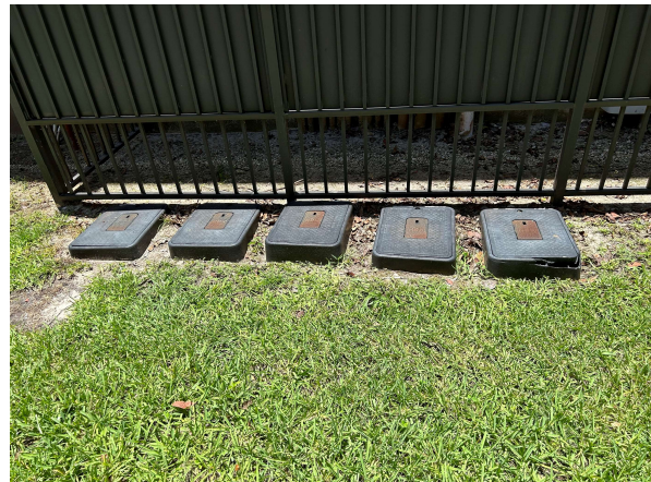
Phase II (Water meter boxes) (22)
