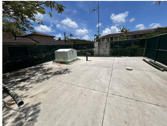
Phase II (Lift Station) (24)
