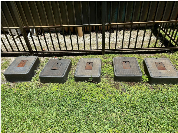
Phase II (Water meter boxes) (21)
