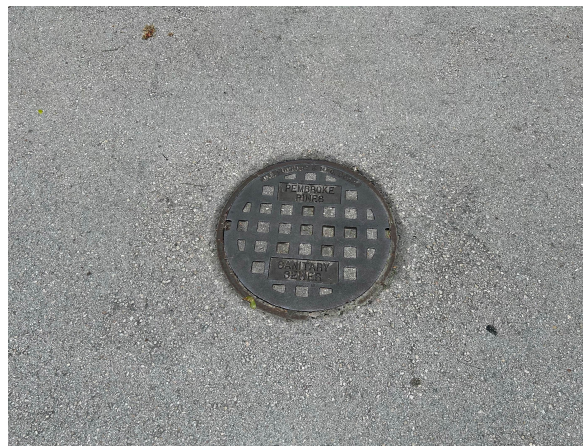
Phase II (Sanitary Sewer Manhole) (26)
