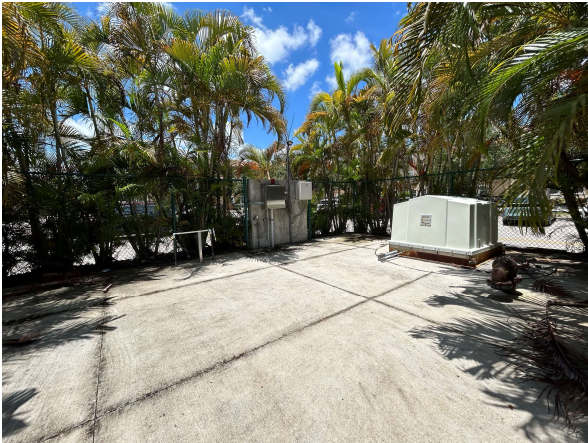
Phase I (Lift Station) (23)
