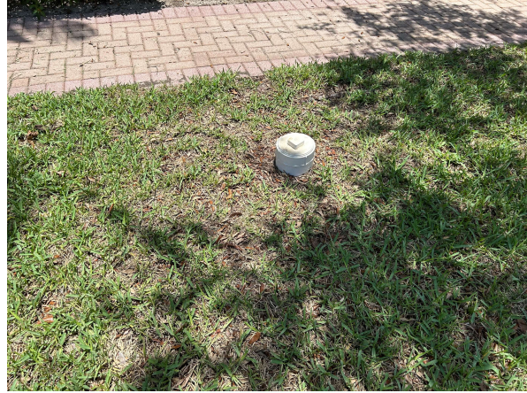
Phase II (Cleanout) (28)
