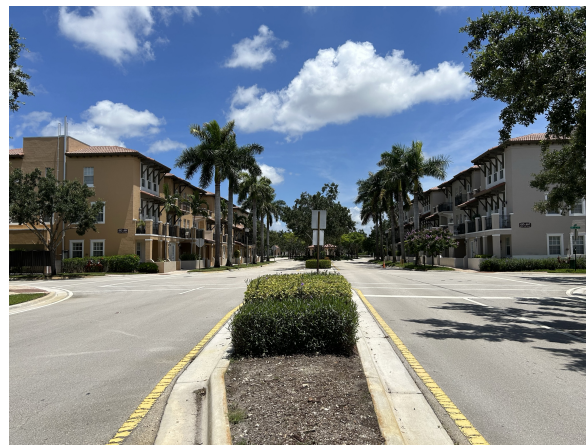
Phase I (Roadway) (2)
